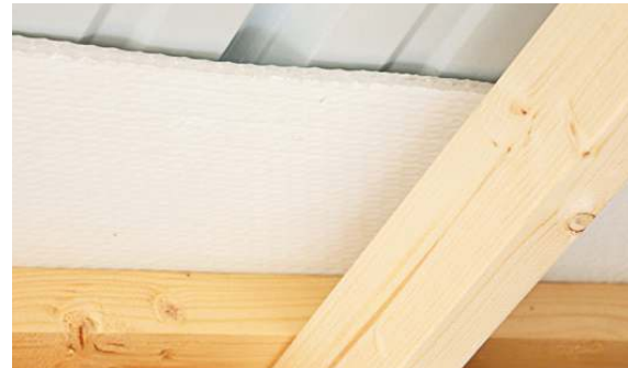
Insulated Ceiling Standard on Metal Roof option
