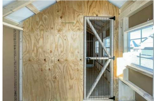
Solid plywood wall with screened door
